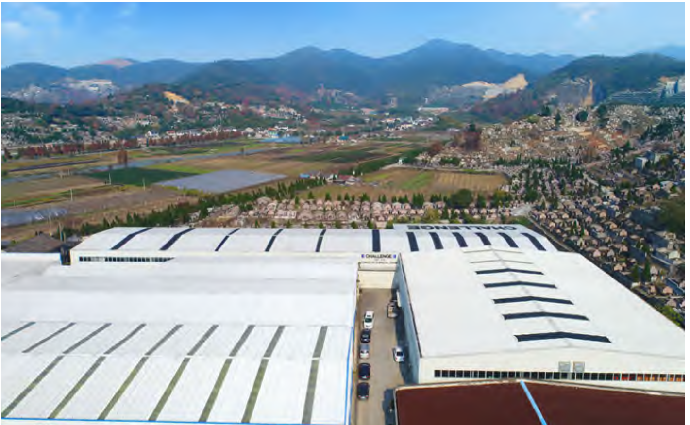
Challenge production plant and warehouse
