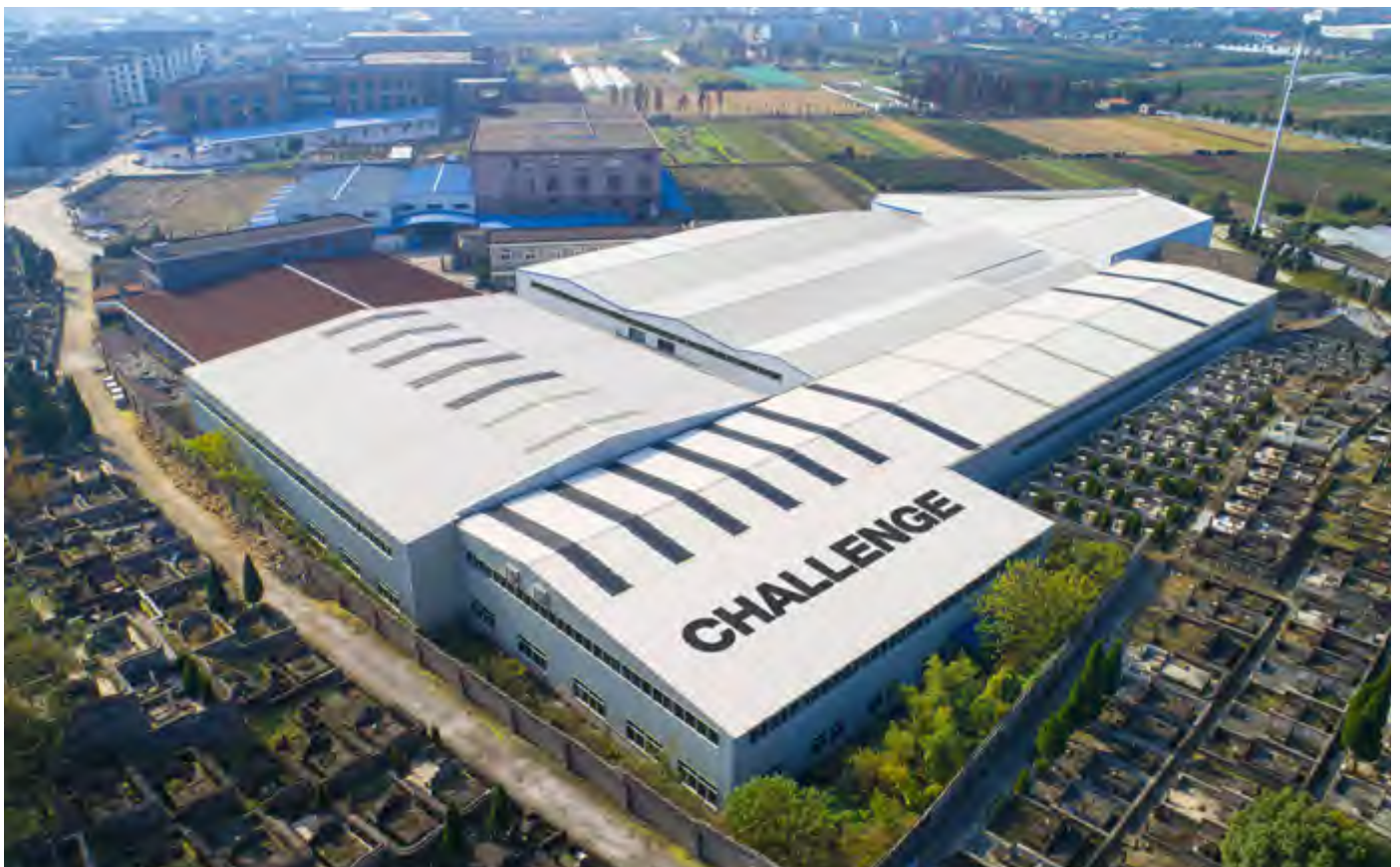
Challenge production plant and warehouse
